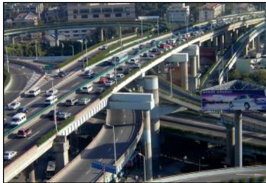
Figure 14. Modern flyover in Shanghai. Photo taken by L. Schipper (2004).
